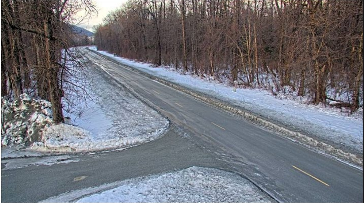
Figure 13: RWIS station at Milepost 23.8, Chilkat River Bridge, Haines Highway (Retrieved February 10, 2026)
